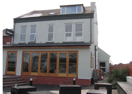
Completed Front Elevation
